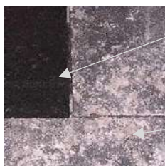
Fig. 56: Fire-brick floor parts
